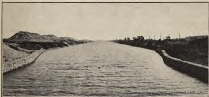
2. A section of the canal where it passes from the solid rock to the soft earth.
